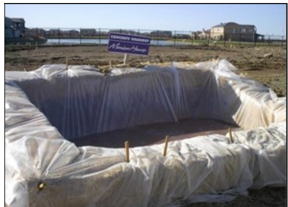
Self-installed washout container with 10-mil min. plastic.
