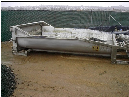
Prefabricated – reusable washout structure.
