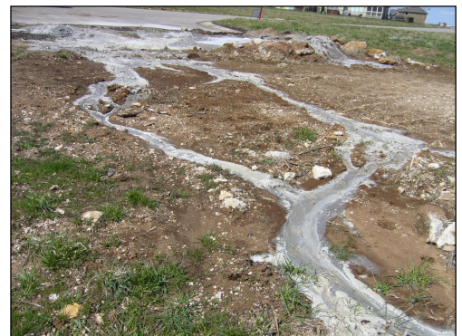
Unacceptable: Pit full and overflowing.
